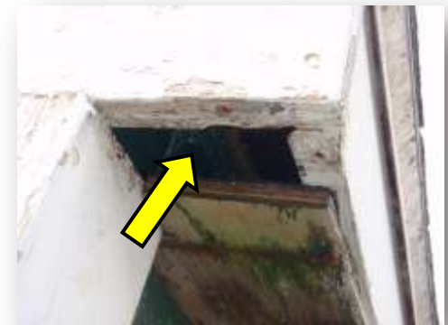
A missing piece of wood on the underside of this soffit makes it easy for birds or squirrels to enter
