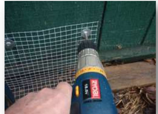
Attaching hardware cloth using a cordless drill/driver, lath screws and fender washers
