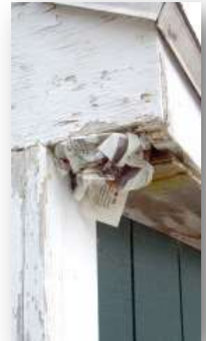
After starting hazing techniques (see text), a loosely-packed ball of newspaper stuffed in an animal's entrance hole can help you tell if an animal has moved out or not.
