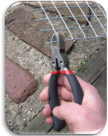
*Trimming welded wire mesh with a wire cutter. Wear safety glasses when cutting mesh*
