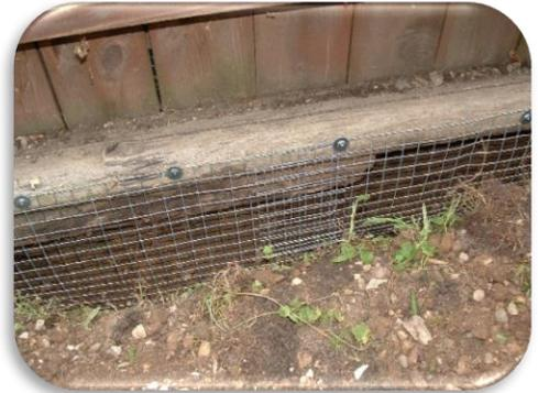
*Welded wire mesh in a trench dug next to a fence that forms one side of a deck. The mesh is screwed to the deck using lath screws and fender washers. The trench is then back-filled with soil*
