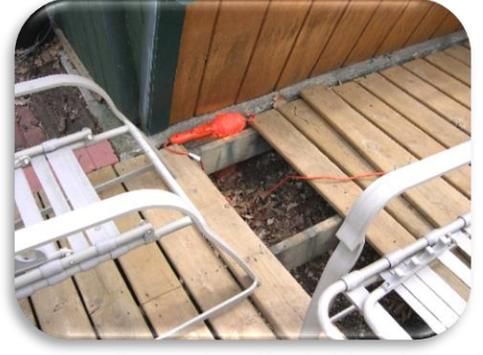
Temporarily removing a few deck boards over the location an animal likes to sleep can encourage it to give up on that location. Adding a light source like the trouble-light shown here (arrow) may provide additional incentive for the animal to move out. Be sure to cordon-off the area so someone doesn't step into, or fall into, the opening.
