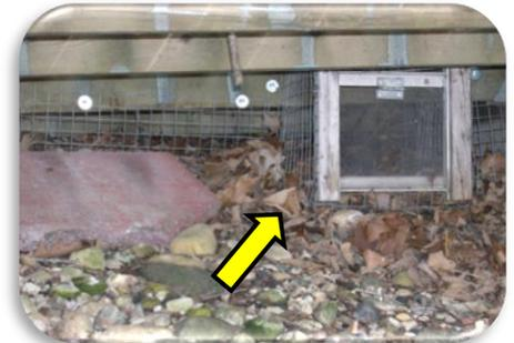
*A one-way door (arrow) and exclusionary mesh installed on an opossum entry under a deck built on a slope*
