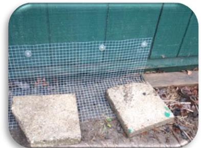
*Trenching was not possible here, so the "L"-shaped mesh barrier is left above-ground. The mesh will be buried under rocks or soil*
