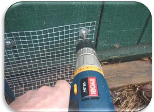
*Attaching hardware cloth using a cordless drill/driver, lath screws and fender washers*
