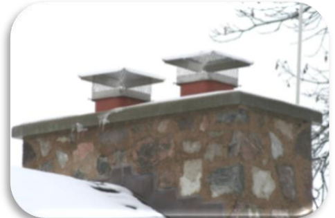
These chimneys have had sturdy, stainless steel chimney caps installed
