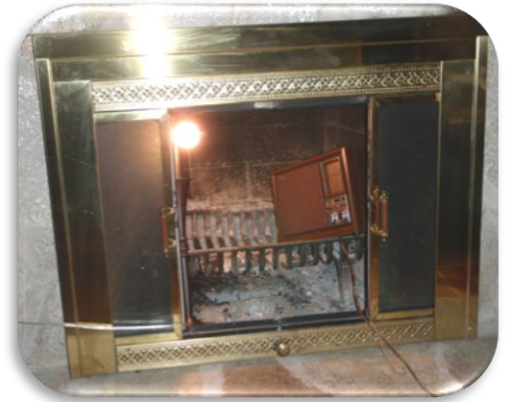
A bright table lamp with the shade removed and a portable radio placed in the fireplace to try get a raccoon to move out of a chimney
